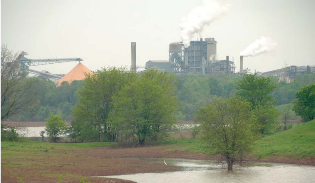
Green Bay Packaging, located along the banks of the Arkansas River in Morrilton, Arkansas, has two linerboard machines that produce corrugating medium and linerboard grades ranging from 26 lbs to 69 lbs.
